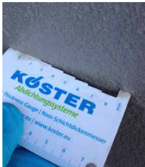
Picture above: Checking the layer thickness of KÖSTER NB 4000 waterproofing.
