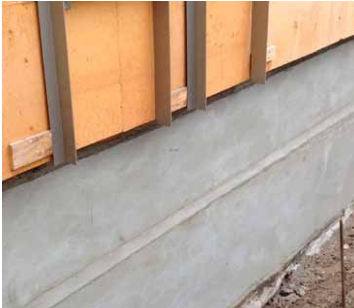
Picture above: prepared substrate; picture right: application of KÖSTER NB 4000.
